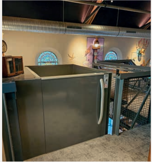
The lift has a 1.1-metre-high gate on the top floor that makes the limited space of the mezzanine feel both open and airy.
