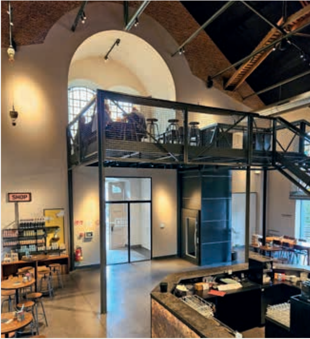
The resto-bar of the micro-brewery is equipped with a Cibes A5000 platform lift to facilitate access to the mezzanine floor.
